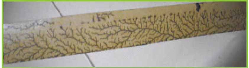
Tracking traces on paper insulation of a 150 kV cable
